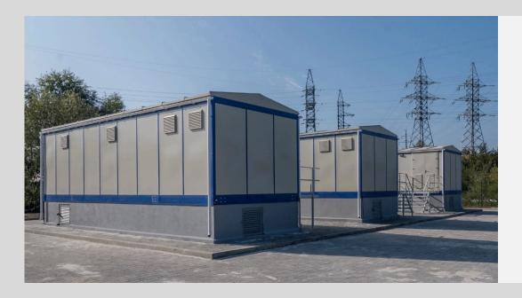
Modular traction substation is a functionally finished product with organization of power and secondary circuits connections.
